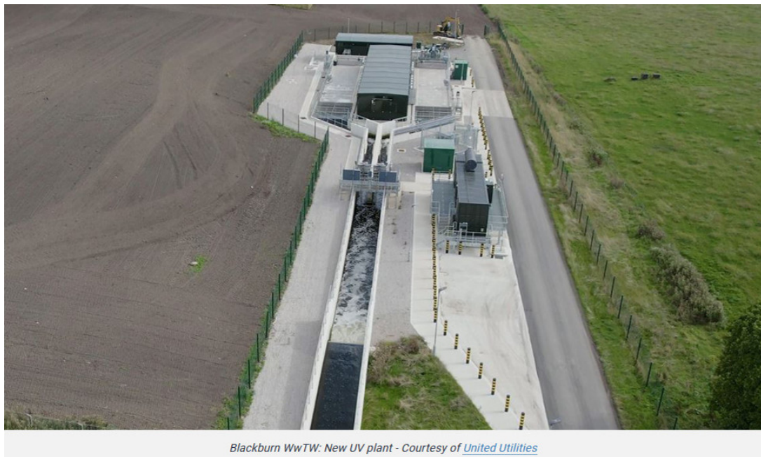
Figure 31 – Aerial view of the Blackburn WRC additional tertiary treatment installation
